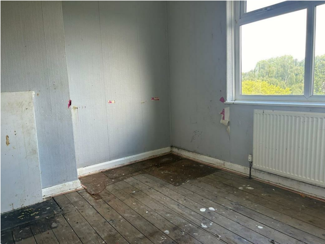
Double glazed window, central heating radiator
